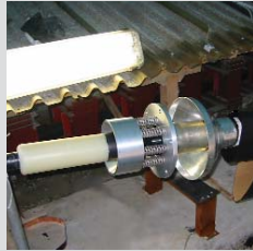
TERMINATION READY FOR TOP CONNECTOR INSTALLATION
