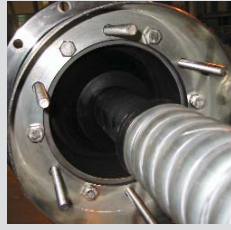
STRESS CONE POSITIONING
